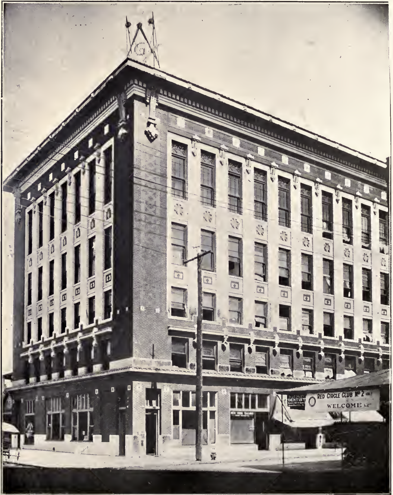
MASONIC TEMPLE BUILDING—JACKSONVILLE, FLA.
