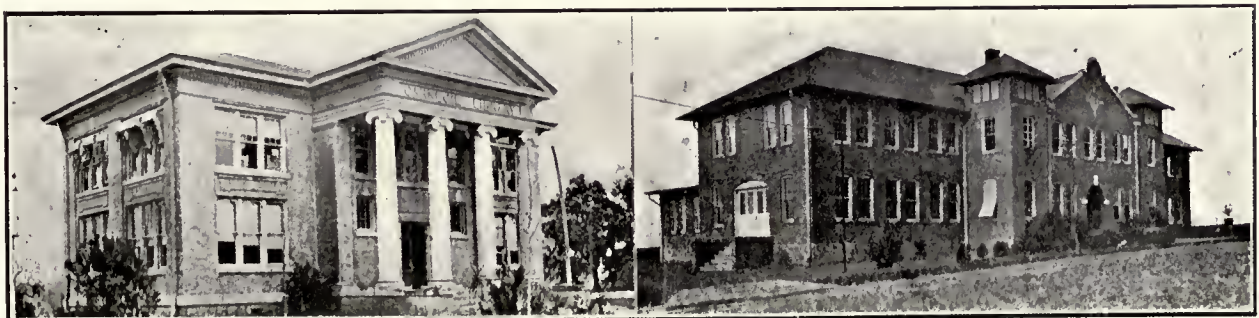
CARNEGIE LIBRARY, STATE A. & M. COLLEGE, TALLAHASSEE, FLA., MECHANICS ART BUILDING
