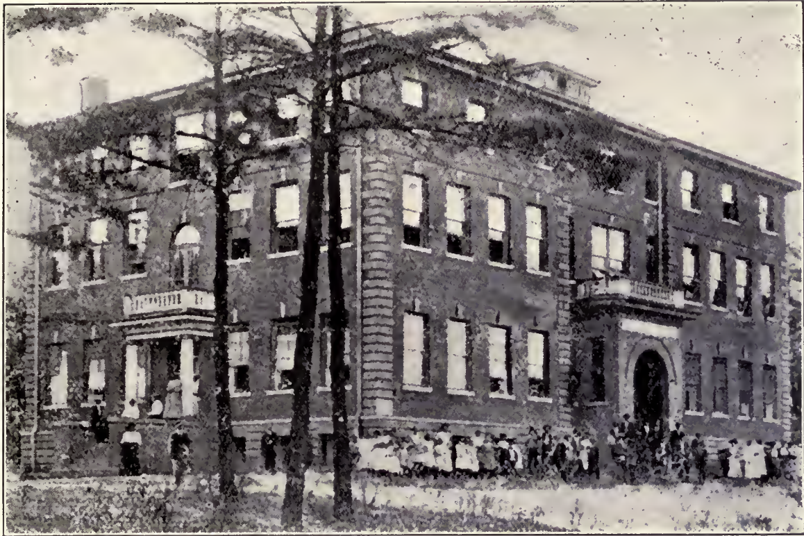
MAIN BUILDING—CENTRAL ALABAMA INSTITUTE
