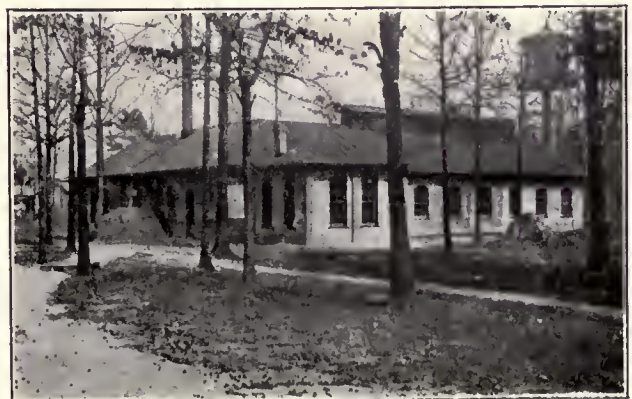
MECHANICS ARTS BUILDING—BRANCH NORMAL COLLEGE
