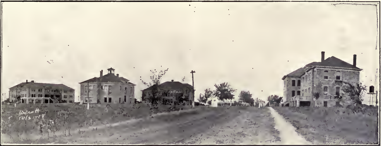
PARTIAL VIEW OF CAMPUS—INDUSTRIAL AND EDUCATIONAL INSTITUTE.
