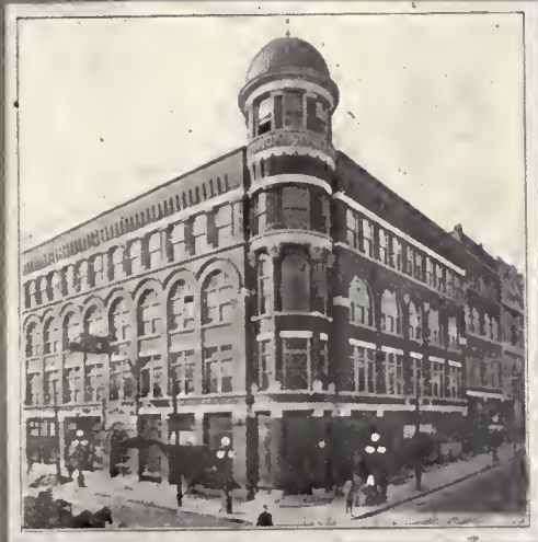
Y.M.C.A. BUILDING, NASHVILLE, TENN.
