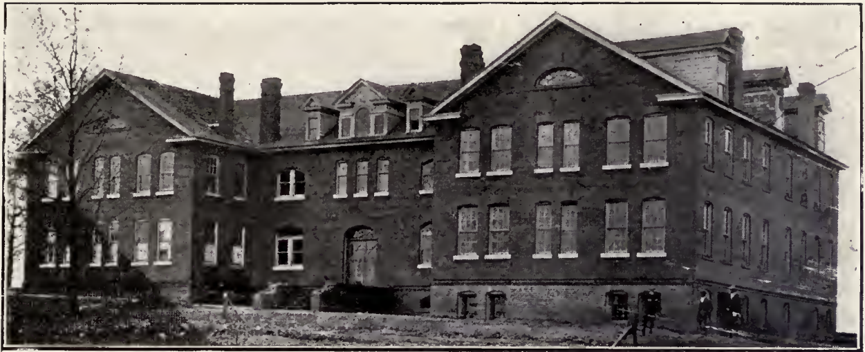
BALLARD INDUSTRIAL BUILDING—LIVINGSTONE COLLEGE
