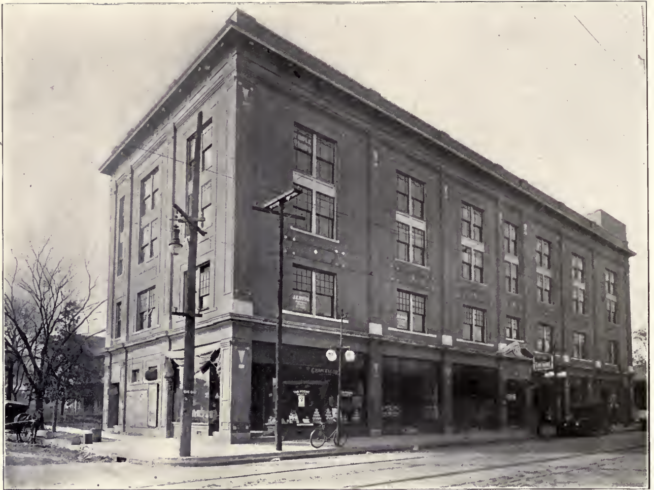
MOSAIC TEMPLARS' OFFICE BUILDING, LITTLE ROCK, ARKANSAS.
